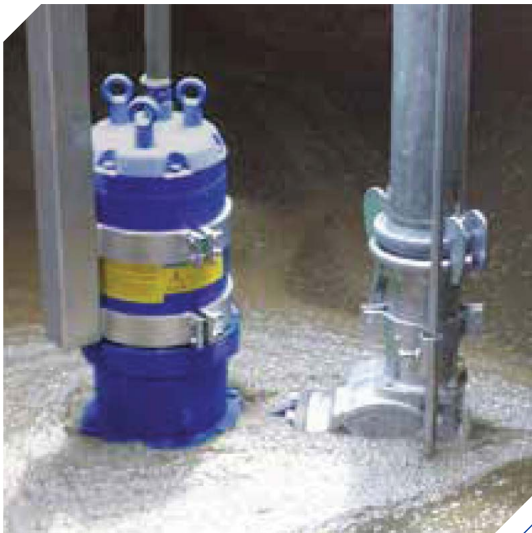
FEEDING OF THE SYSTEM WITH A SPECIAL SUBMERSIBLE MOTOR CHOPPER PUMP
